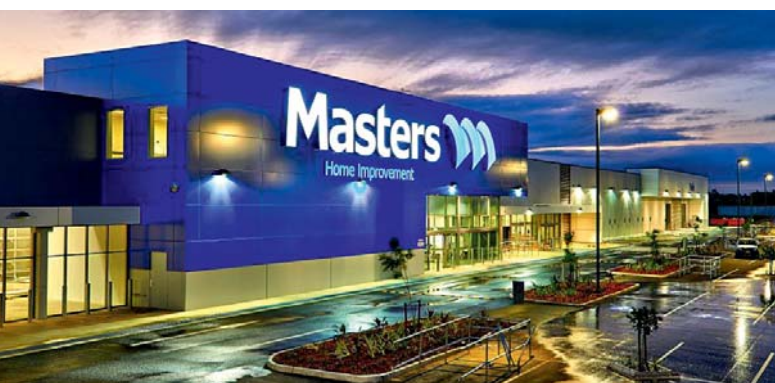
HUTCHIES has finished work on the first Masters Home Improvement centre in Mackay. Built at a cost of more than $14 million, the centre consists of 13,000m 2 of floor space with a dedicated garden centre and a 373-space carpark.
