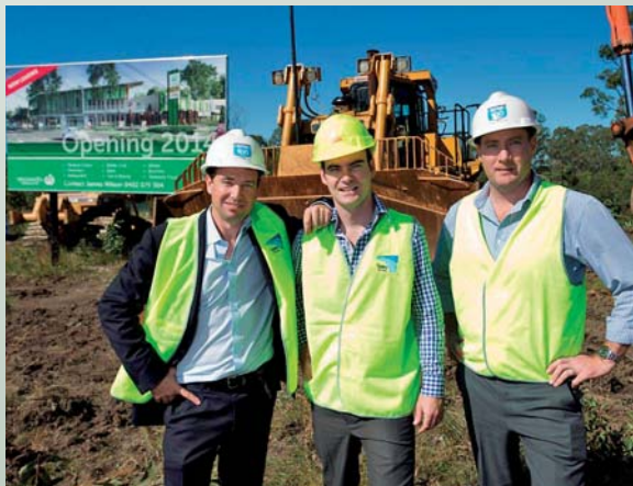
From left, Woolworths regional property manager, Phillip Peel; Tipalea Partners managing director, Scott Spanton; and Hutchies' project manager, Russell Fryer, at the Pimpama Junction ground-breaking ceremony.
